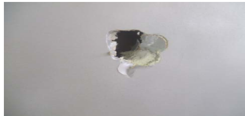
Figure 1. Damaged Gypsum Board
