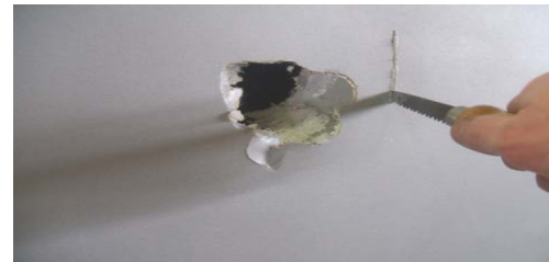
Figure 2. Square-Off Damaged Area
