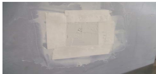
Figure 5. Tape and Finish Patched Area
