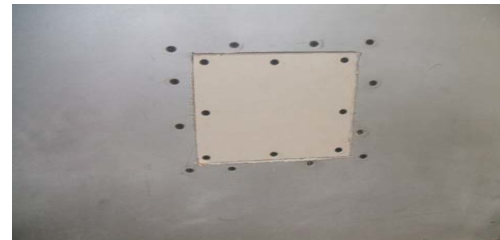
Figure 4. Apply Gypsum Board Patch
